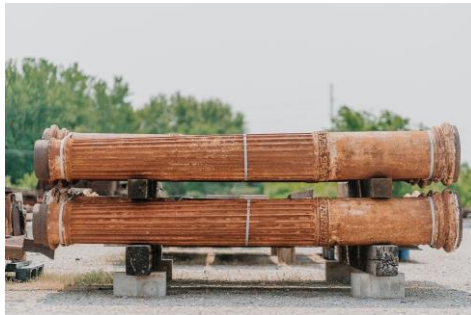
Cast Iron Column, Clemens House, 1860
